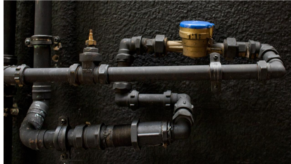
Pipe with “minor losses” components
